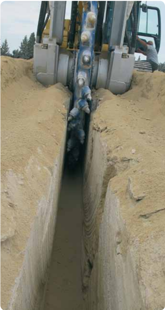
ERW 1000 trenching in medium hard limestone
